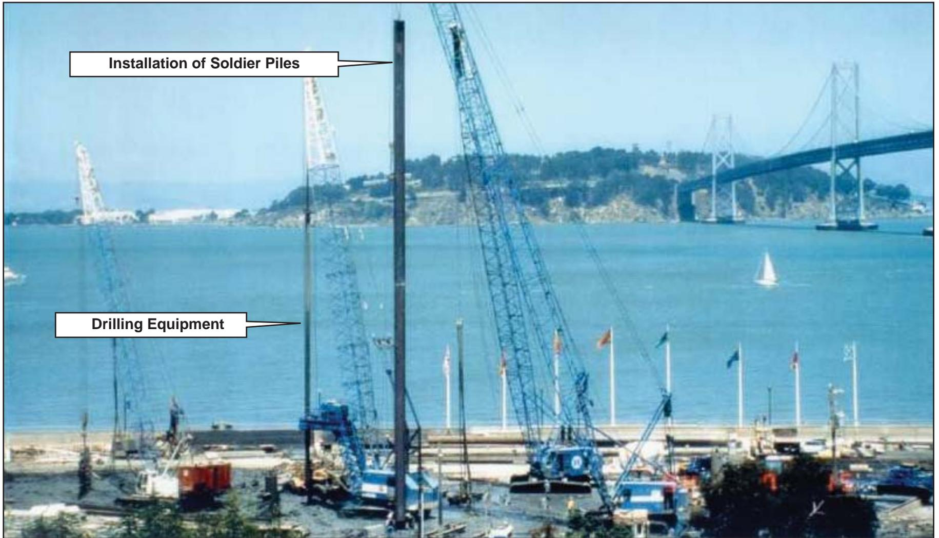
**FIG\_196: Installation of Soldier Piles for SPTC Wall**
